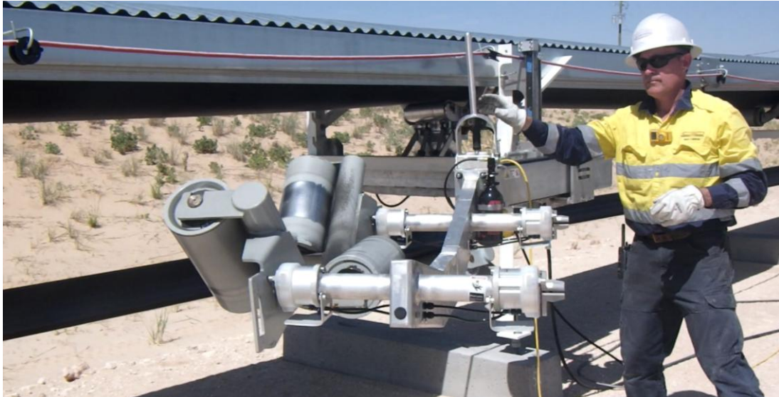
Figure 8: Idler Transom frame and roller assembly being reinserted
