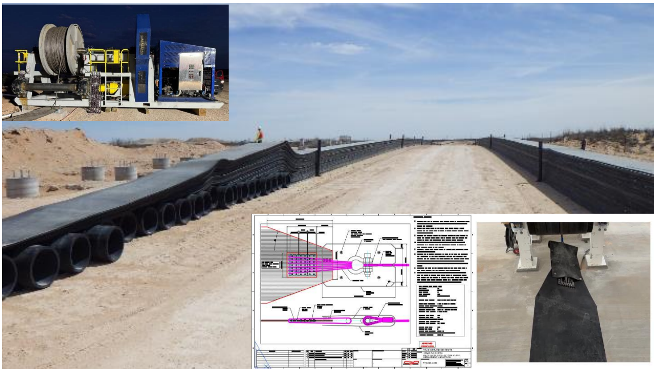
Figure 3: Pre-spliced belt flake stacks up to 20.7 km in length with custom belt pulling plate and 4.5 km cable winder capacity
