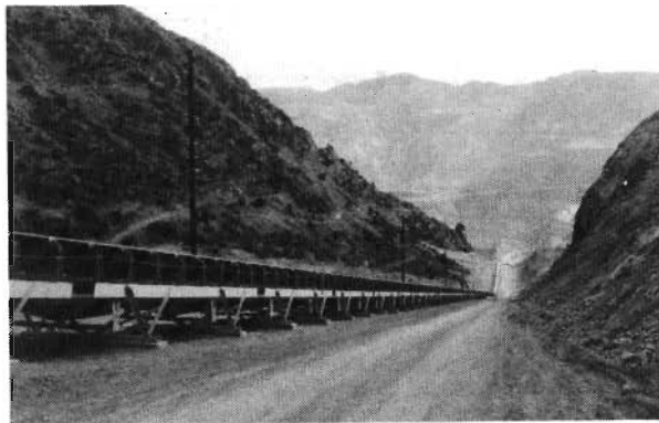
Figure 3 The P7 downhill conveyor at the Phelps Dodge Morenci copper mine in Morenci, Arizona, has 245 meters of drop and uses inverter drives and hydraulic disk brakes.
