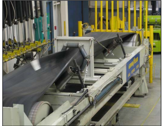
Figure 3. Pipe belt transition test.
